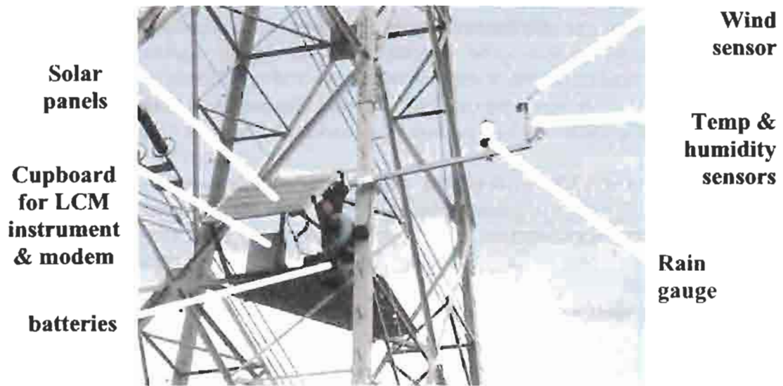
Fig.4: The components of a LCM test station (1)
